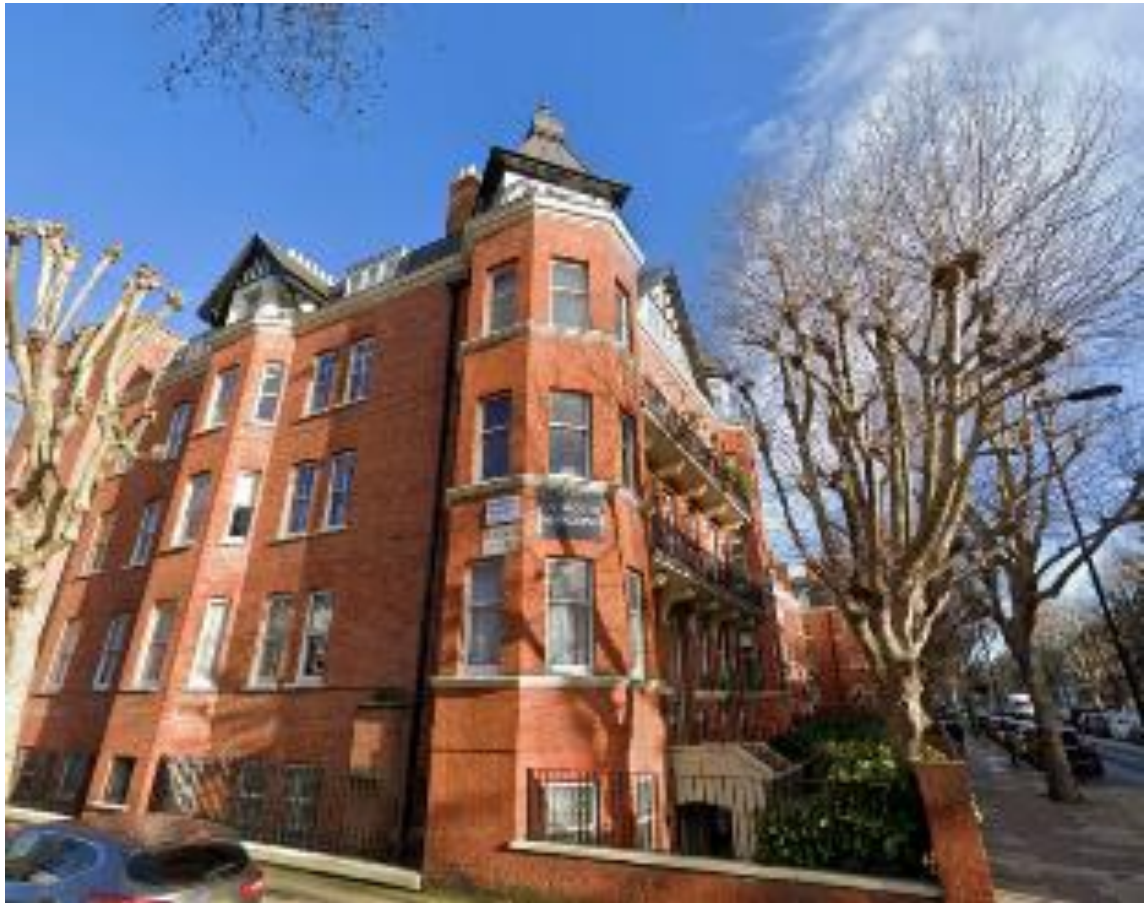
Front Elevation; Flat 44 is at 2 nd Floor with the windows on the corner.
